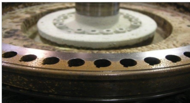
FIGURE 2. RUSTED UPPER TURRET SECTION
