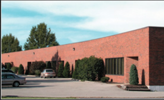
TURRET MANUFACTURING FACILITY CHESTERFIELD, MISSOURI, USA
