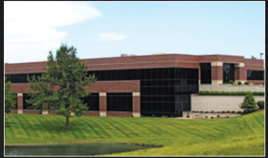
TECHNICAL TRAINING & PRESS REFRUBISHING FACILITY ST. CHARLES, MISSOURI, USA
